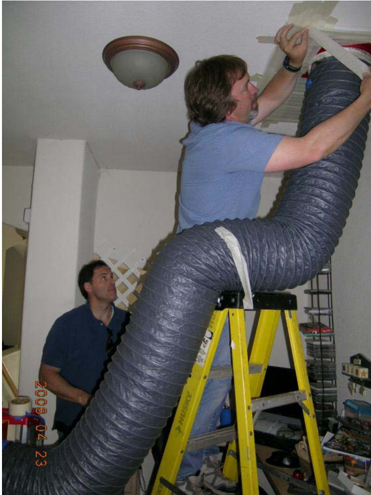
Attaching to a ceiling return.
