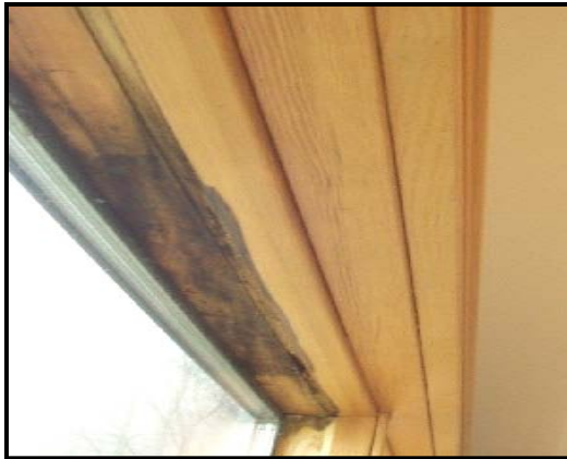
Top Sash after trim removed
