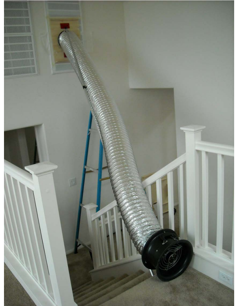
Attached to a wall return.
